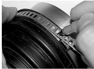
Step 2 Determine the clamp length.
