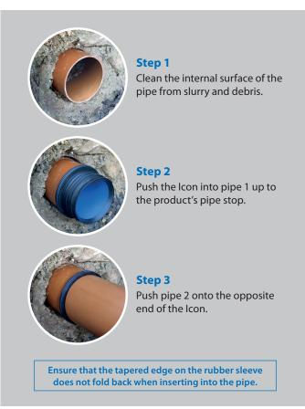
Note: The lip in the rubber is tapered to eliminate steps in the joint and aid natural flow. Not suitable as a pipe support. Bored reduction has been kept to a minimum and is deemed suitable for drainage applications; the coupling has specific design features that help to keep the joint resilient to the very small increases in internal pressure over the width of the coupling.
